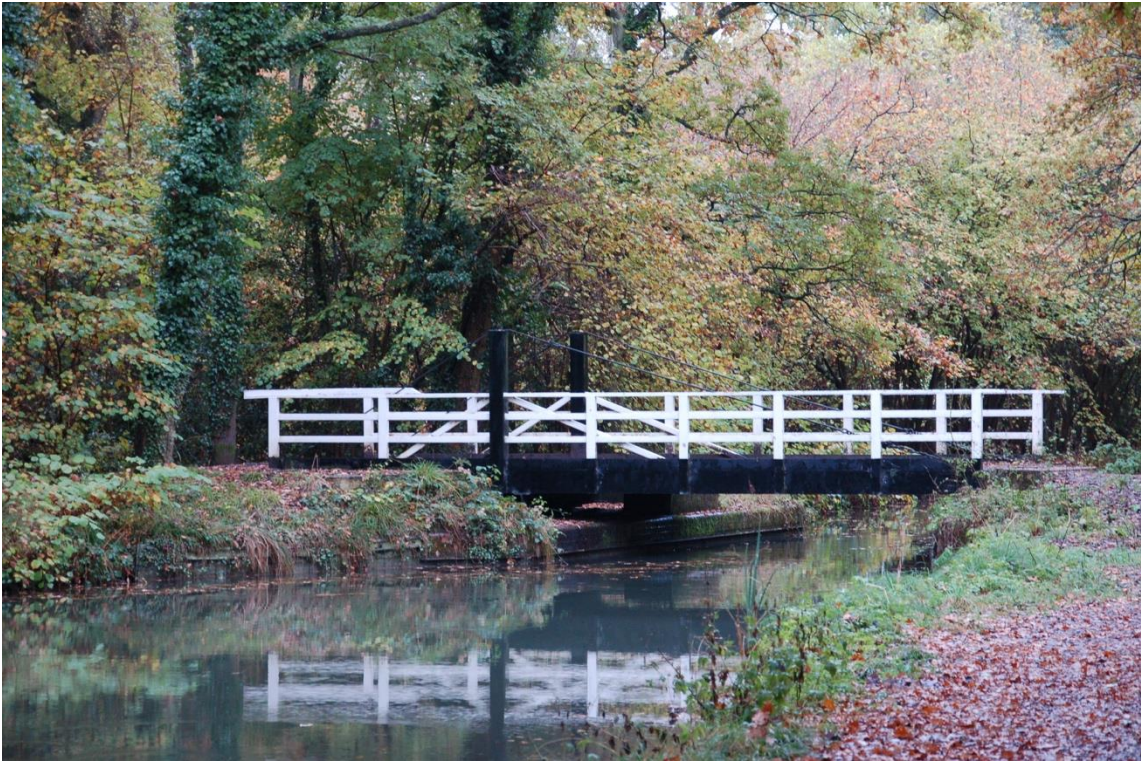
Figure 15 - The Swing Bridge
